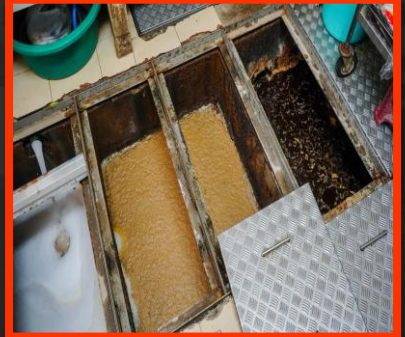
Grease Trap & High Pressure Drain Cleaning
