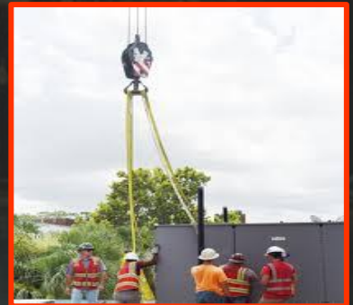
Equipment Installation Works
