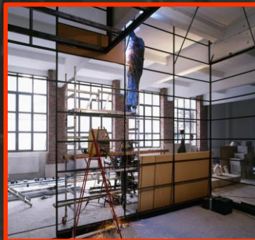
Fit Out Works
