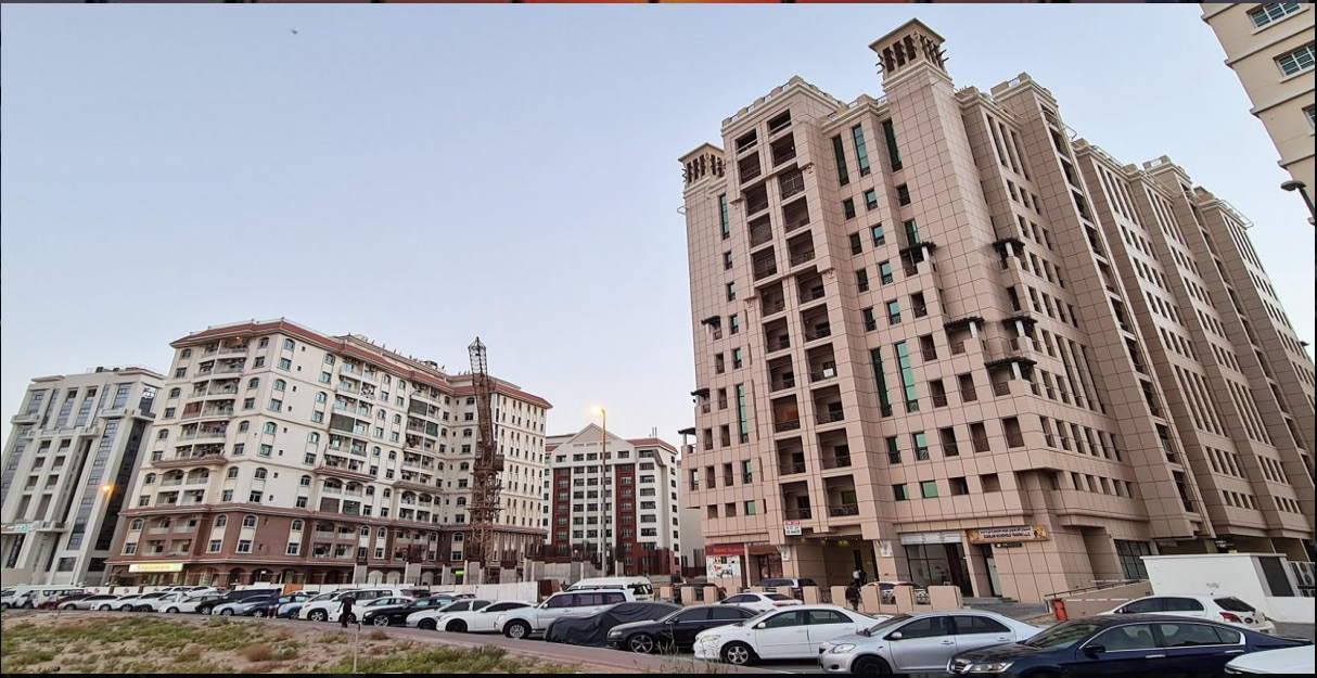
CBD4 Building, Plot No. P-37 , is a mid-rise residential apartment building located at Al Warsan, International City, Dubai, UAE. The property has an estimated built-up area of approximately 180,000 square feet. CHULIA provided annual maintenance services for cleaning, security, swimming pool operations, pest control and water tank cleaning from 2017 to 2022. The building is owned by Real Estate Services .
