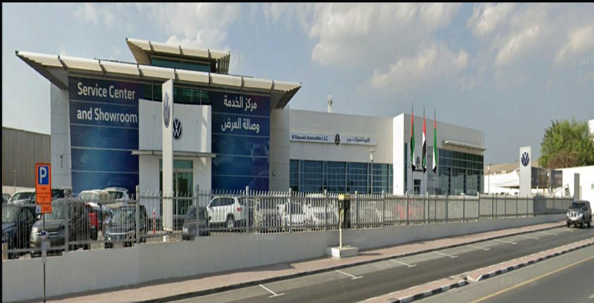
The Volkswagen Service Centre and Showroom at Rashidiya, Dubai, is a combined automotive sales and aftersales facility supporting vehicle display, maintenance, diagnostics and customer service operations. The facility comprises showroom areas, service workshops and support spaces, with an estimated gross built-up area of approximately 120,000 square feet. CHULIA has been the Facilities Management operator since 2015, supporting operational reliability and brand standards.
