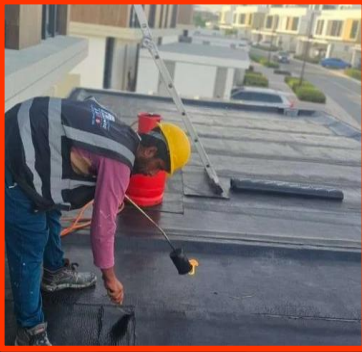
Water Proofing Works
