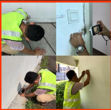
Building Condition Survey
