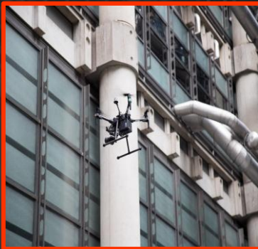
Drone Inspection & Survey
